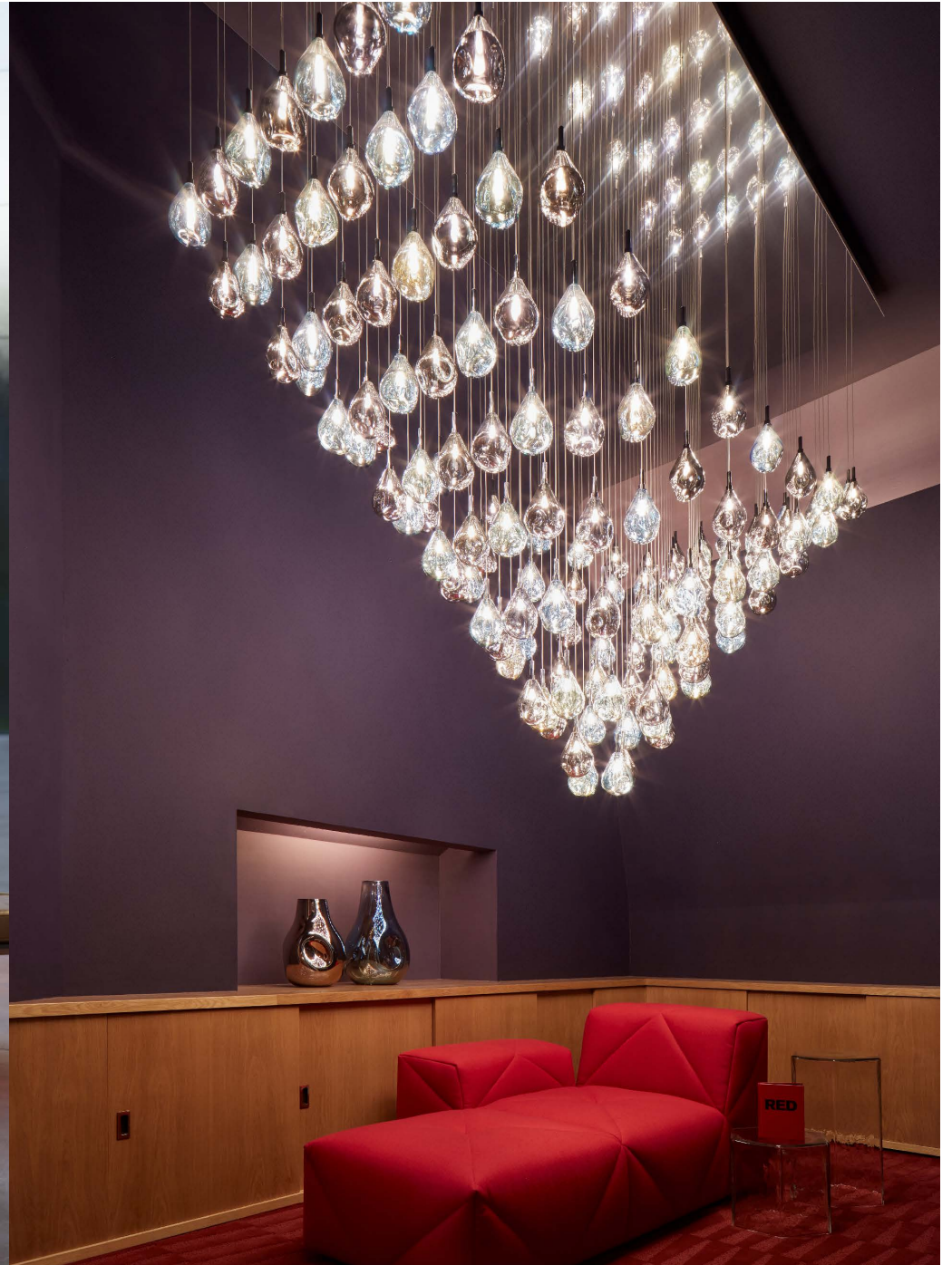
BOMMA Atelier, Prague, 2021 - installation of 142 pcs
